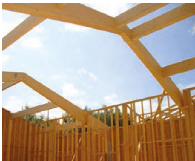
Figure 9 Glulam portal frames
