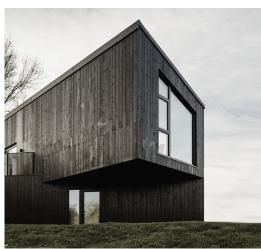
The aim was to create an upside-down house using CLT to create two cabins that merged with the surrounding area and provided an energy efficient and striking design through it's 45 degree offset layout.
