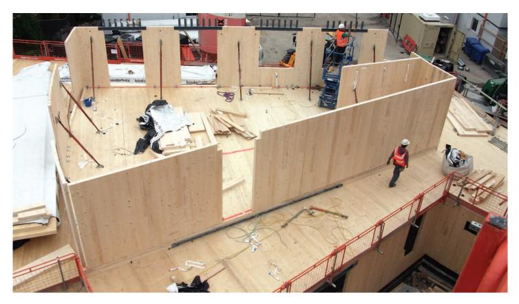
Image 1 - CLT walls and floors during construction
