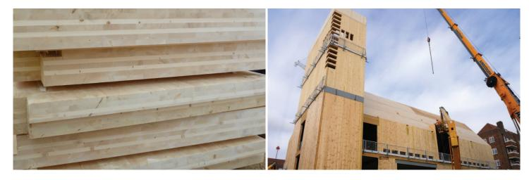
Image 2 - CLT wall slabs
