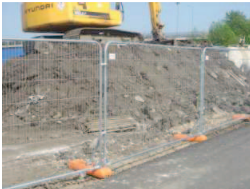
Open mesh type fencing
