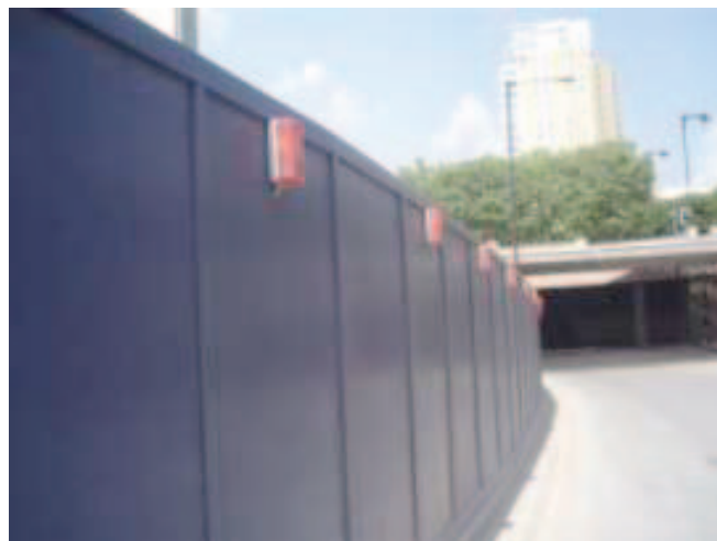
Site perimeter hoarding
