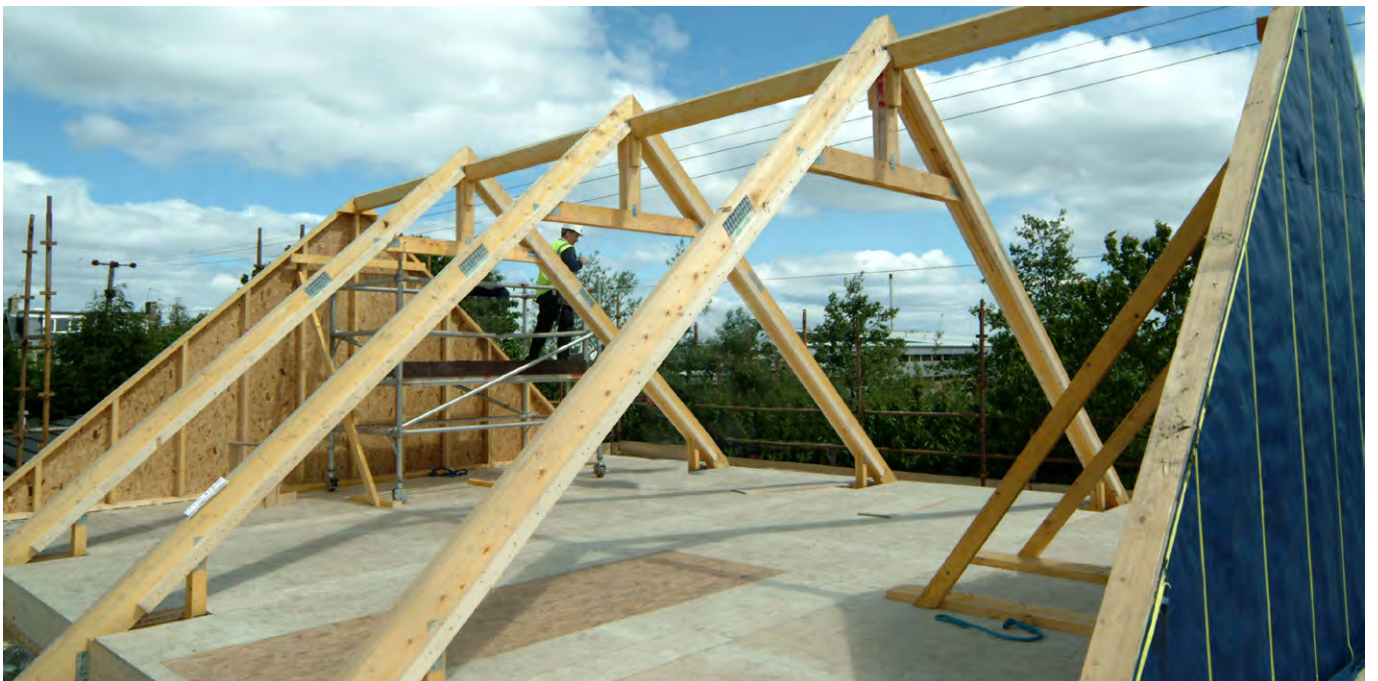
Roof truss construction. Donaldson Timber Engineering
