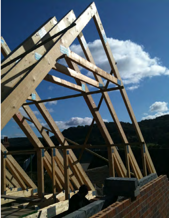
Attic trusses being erected on site.
