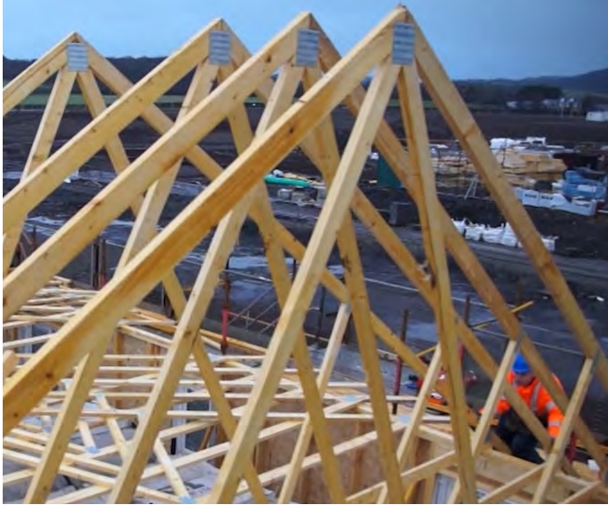
Roof truss erection on site.
