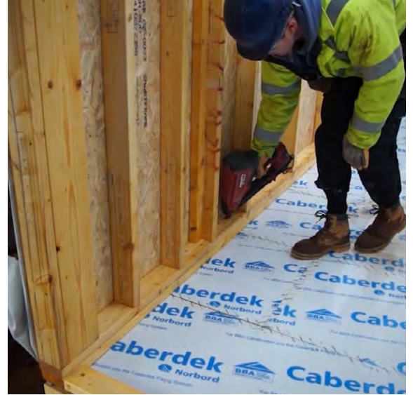
Wall panel erection on site.
